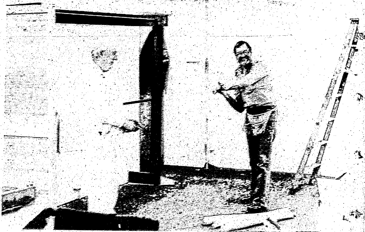
Taking a pause in their remodeling work to recount days of glory on the diamond are Mickey McNeven and Keith Hallman [at bat], who are helping David McNeven prepare a new location for his Coaches Corner.
