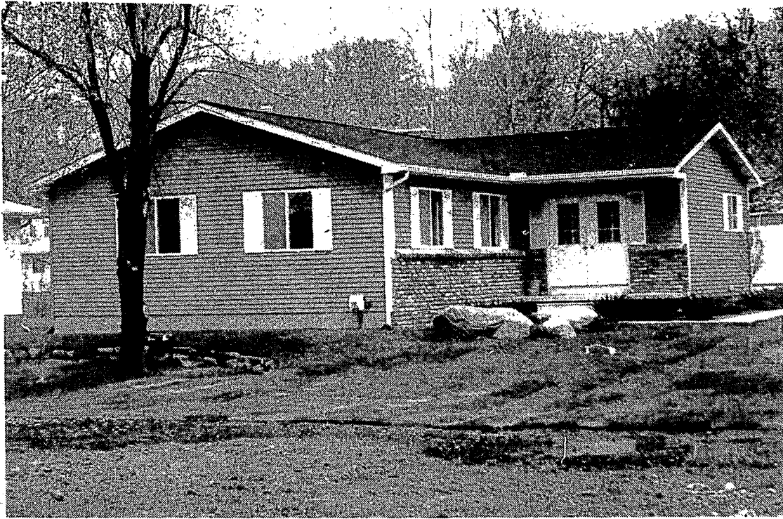
Built by Clarkston High School students registered in the new building trades program, this home at 600 S. Main, Clarkston features three bedrooms, three full baths, a sundeck, two fireplaces, and a finished basement complete with a bar. The home will be open to the public Sunday from 2 to 5 p.m.
