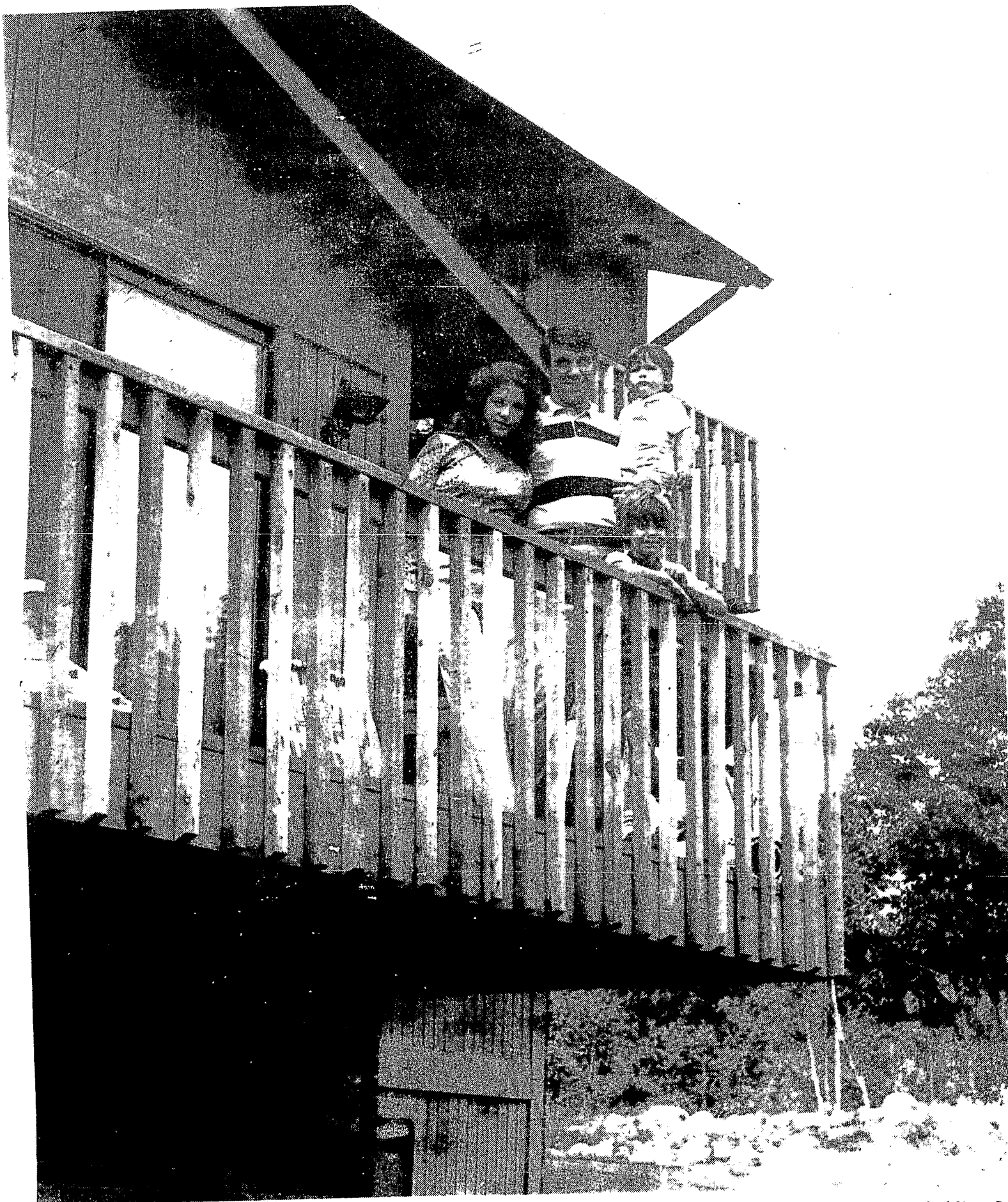
Double decks with spaces between boards made narrow to keep young Scott safe from falling were built on the rear of the Campbells' home by Colin. The decks offer a view of the
