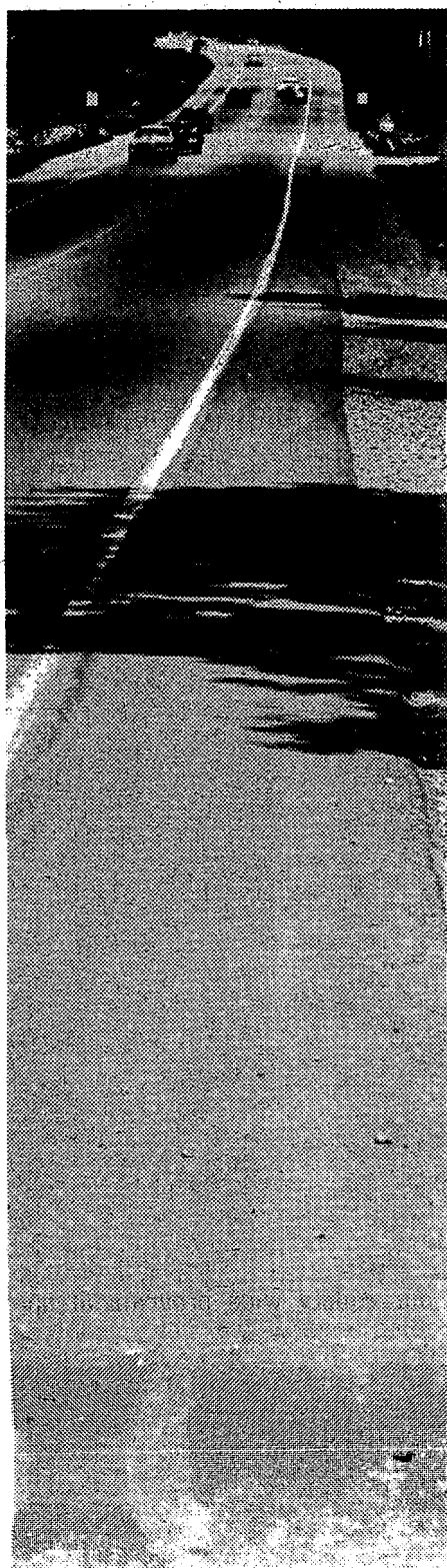
SHOULDER PAVING like this along M-15 will be accomplished in several selected locations on county roads as part of the Road Commission Highway Risk Management hazard countermeasures.
