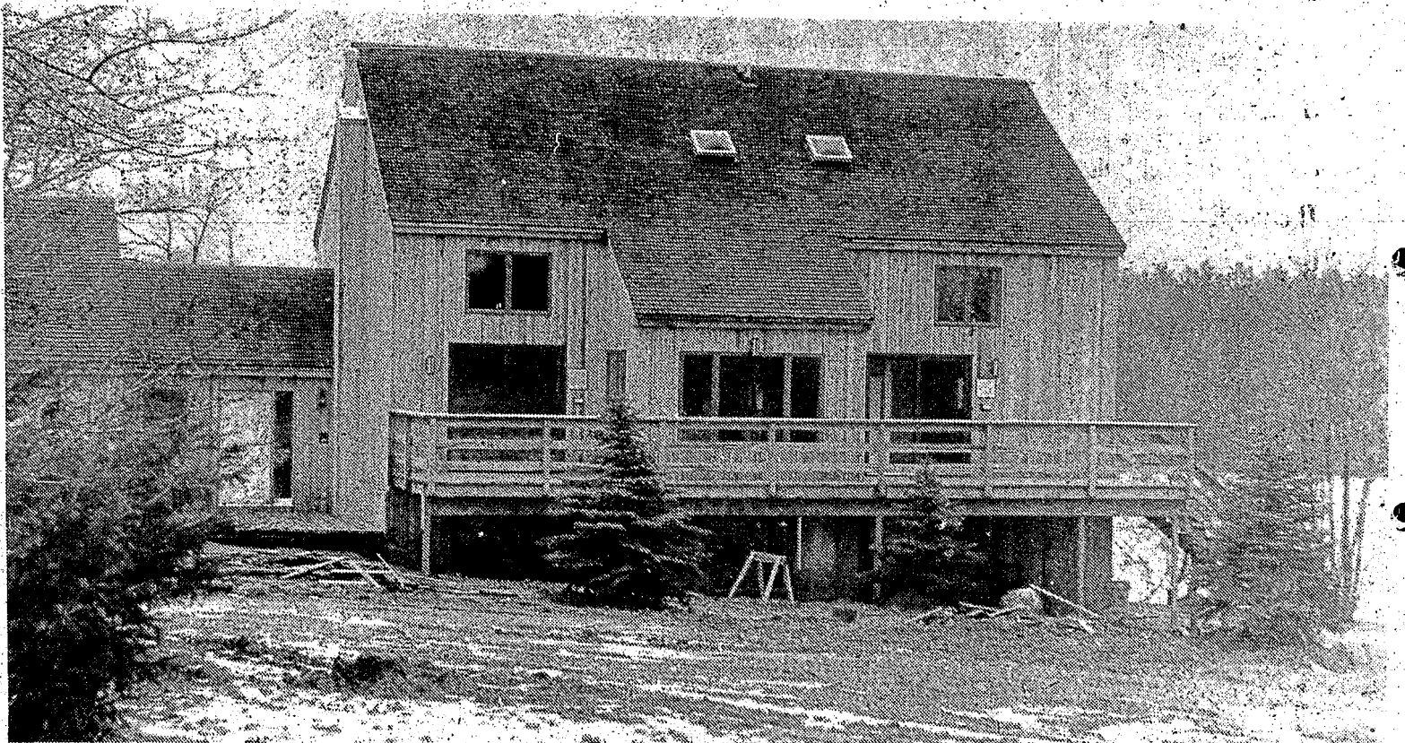
The large windows in the house face south to allow the sun to aid its warmth during cold months. Other energy-saving features include extra insulation, an automatic thermostat with
