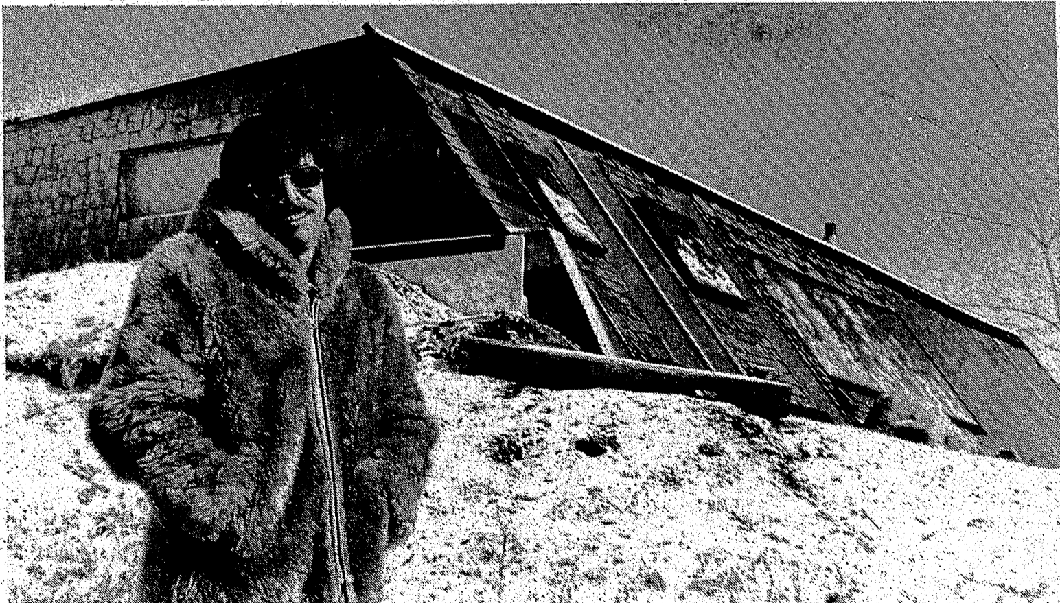
It was 73 degrees inside Jerry Clark's solar-heated home when this picture was taken. Outside, it was about 10 degrees, but bright and sunny. A perfect day to heat using the sun's warm rays. Clark says.
