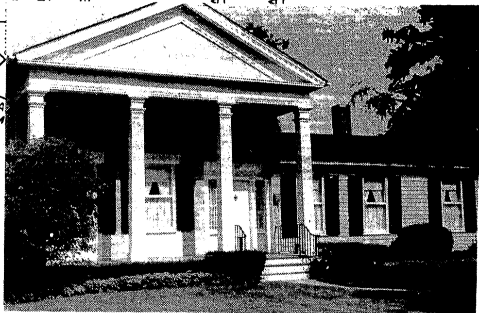
Columns and a full pediment make the Degener home at 58 N. Main a prime example of Greek Revival, circa 1850.
