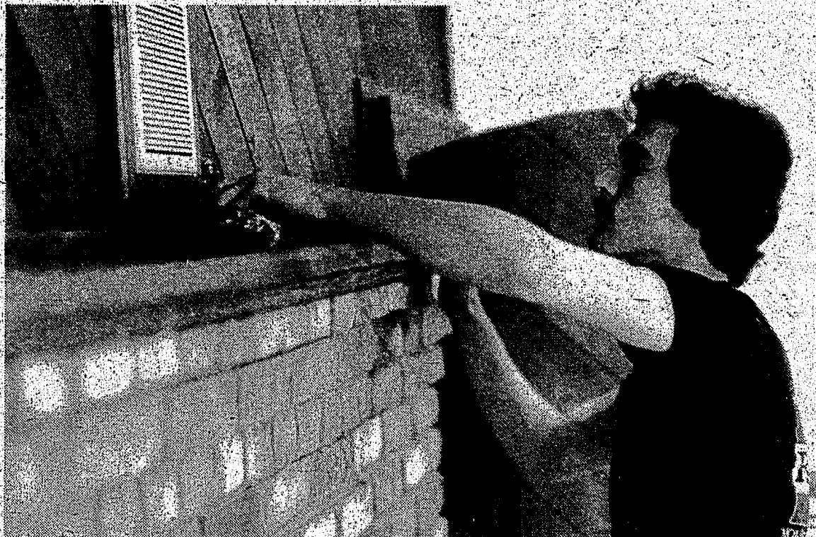
Mike Thompson adds some finishing touches to his work on the heat-saving air vents installed above the large brick fireplace.
