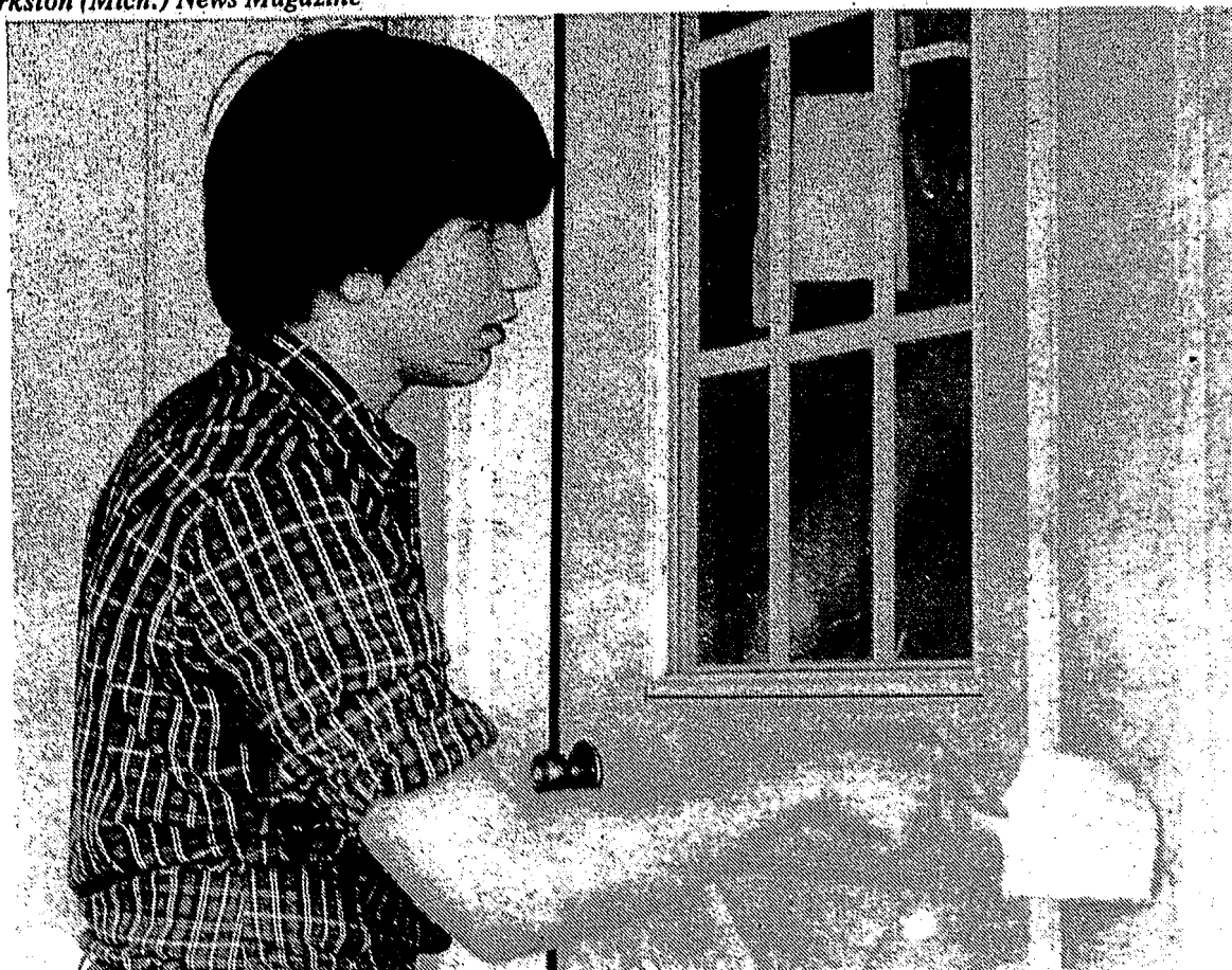
Dale Fulcher spreads the gray paint smoothly and evenly around the frame and wooden walls surrounding the front door.
