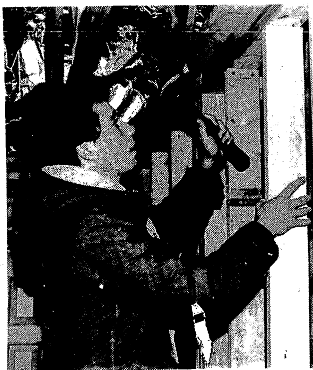
Nailing wall studs is the task at hand for Clarkston High-School's Rod-Hubarth.
