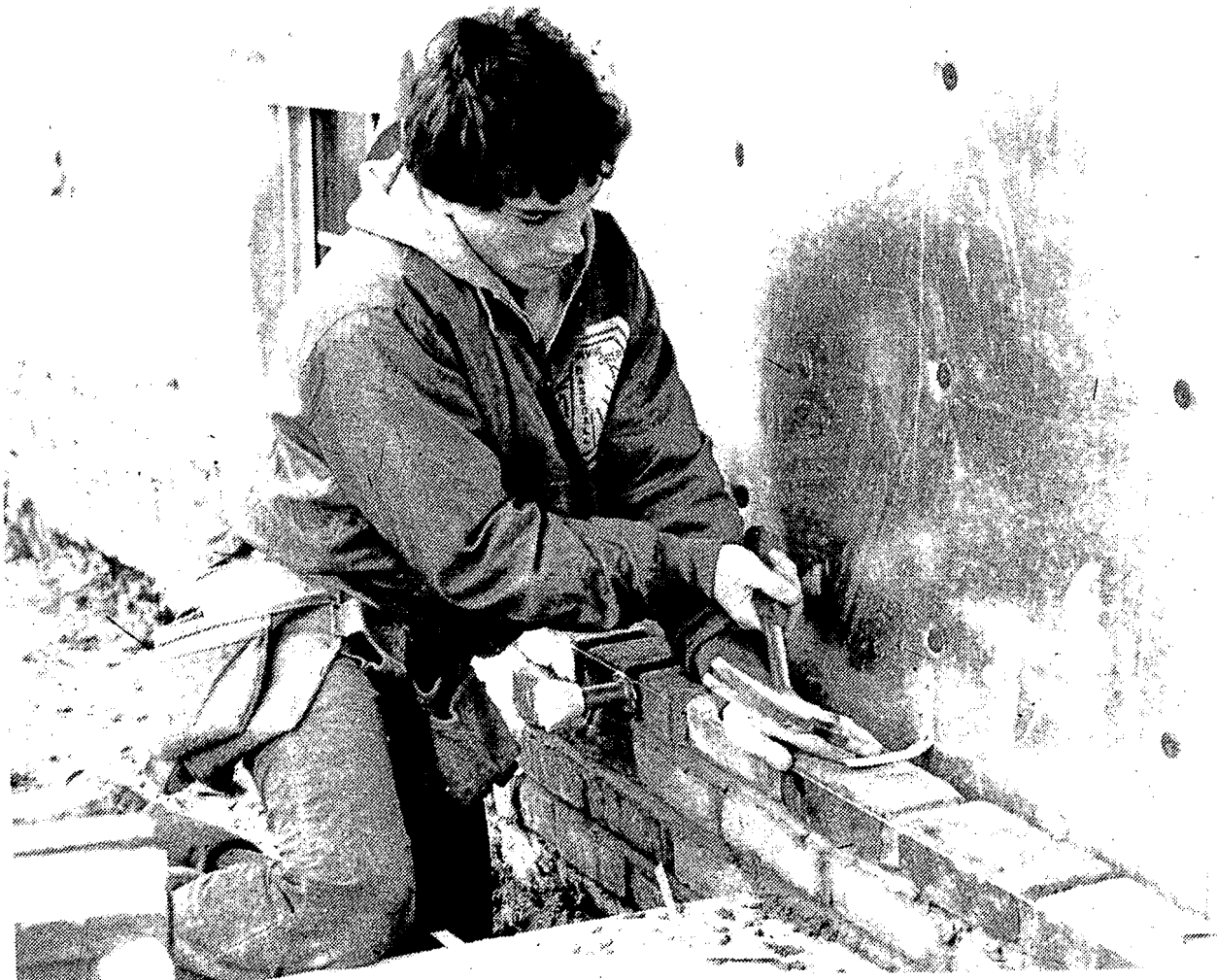
Dave McGeary takes care to securely nail wall ties in preparation for the next row of bricks.
