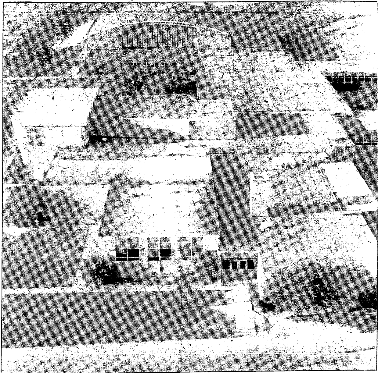
Turquoise accented Clarkston High School, built in 1959 with an addition in 1965, is located on Middle Lake Road and has student body of
