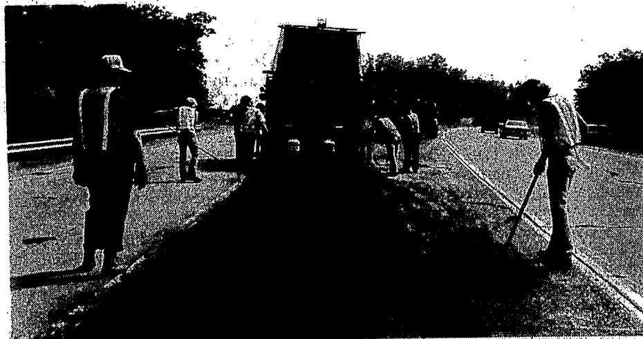
PATCHING — A second machine was added to the Road Commission's arsenal for large-area pavement patching when potholing and edge-rutting reached epidemic proportions after three-years of declining revenues.
