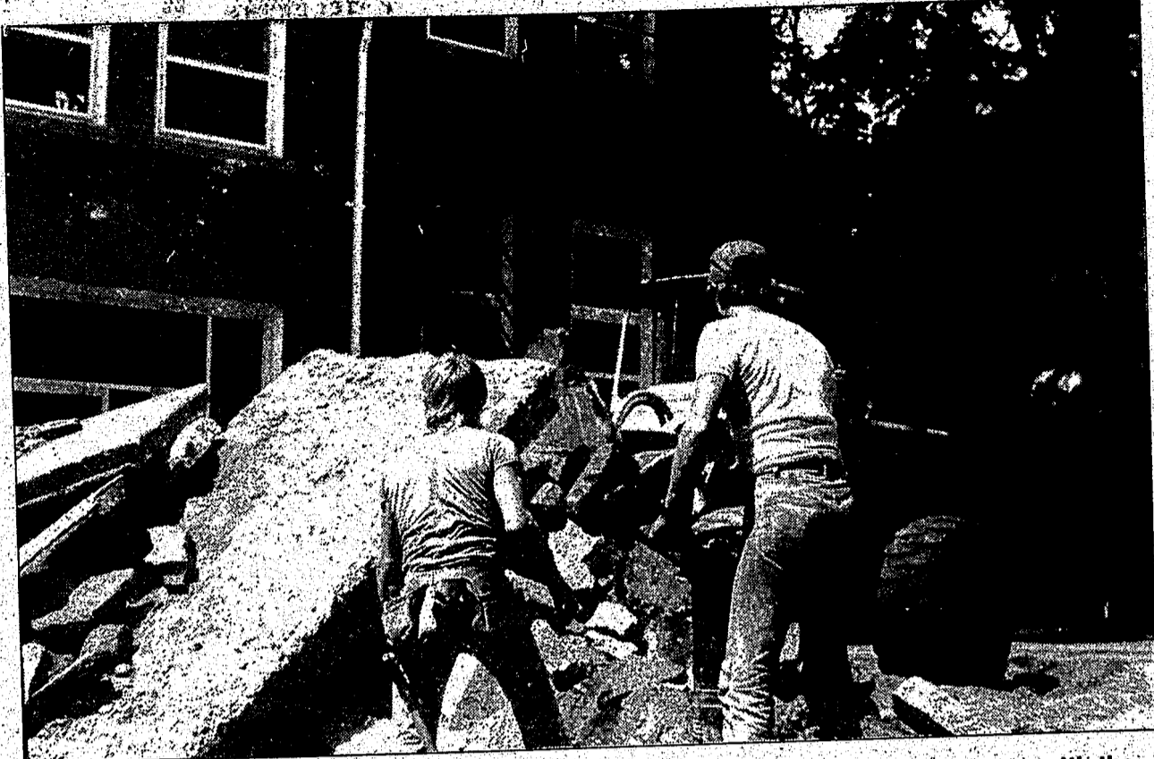
OUT WITH THE OLD: People entering the back of Independence Township Hall Aug. 23 were met by a slight obstruction, a 6-foot-high pile of broken concrete. Workers for Guinn Construction in Pontiac repaired the cement walkway
