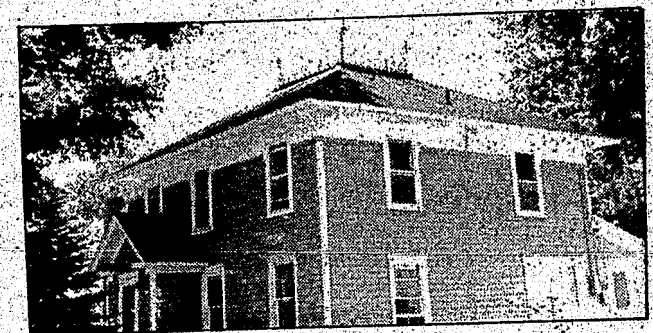
A hip roof on a South Holcomb Road home.
