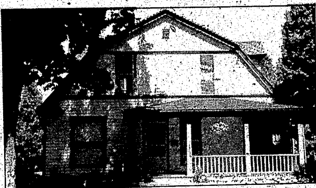
A gambrel roof on a Washington Street home.
