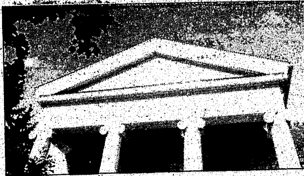
A gable roof on a North Main Street house.
