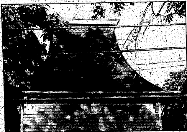
A Mansard roof on a North Main Street home.
