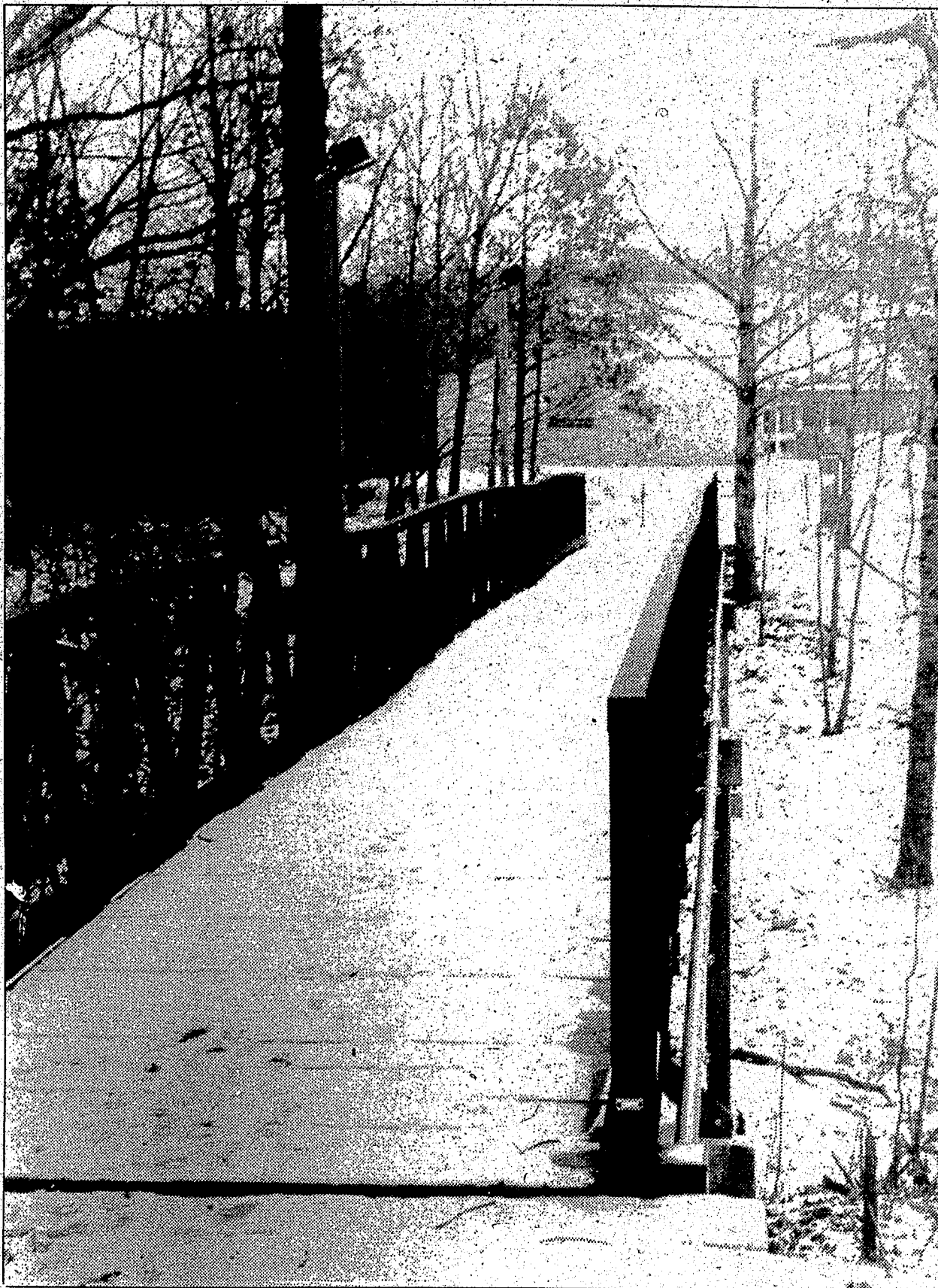
The bridge leading to the nearly completed Nature Center at Independence Oaks County
