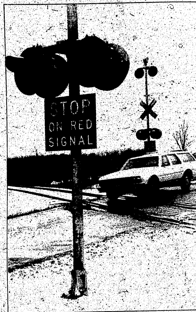
The railroad crossing near Farley Road in Springfield Township is the subject of concern to residents because of loose railroad ties and rough pavement.
