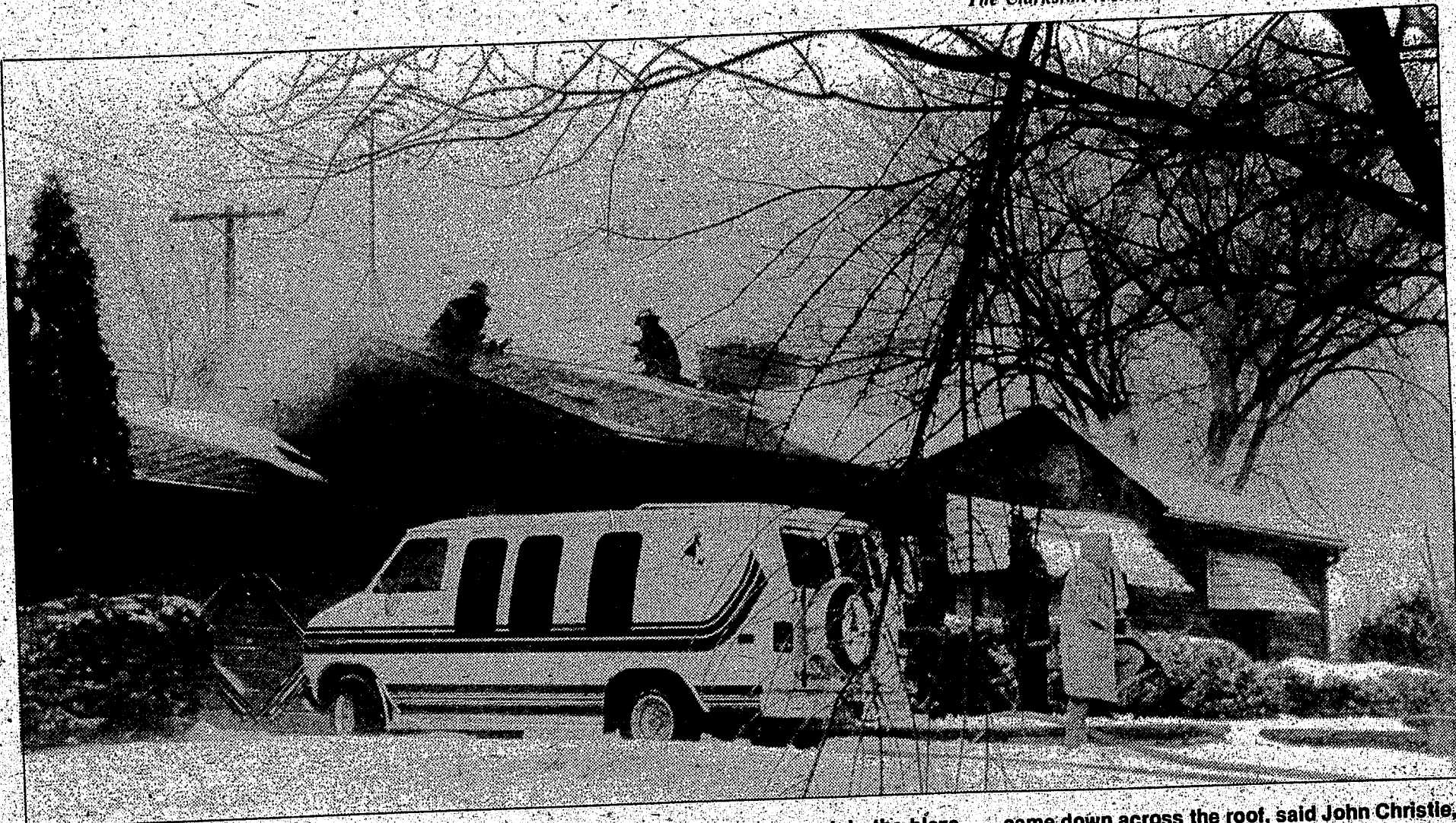
Smoke pours from air vents in the attic of a house on Laurelton in Independence Township while firefighters attempt to contain the blaze. The fire started in the attic when a power line came down across the roof, said John Christie, owner of the home.
