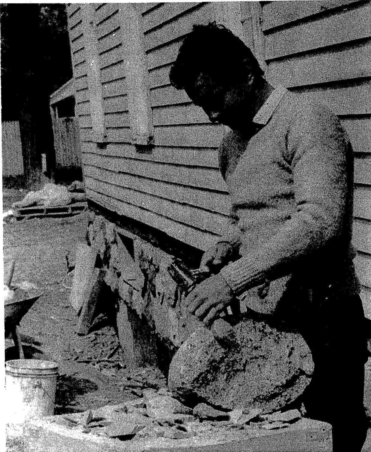
Trimming boulders into rough 5-inch squares for stone masonry is very physical work, but
