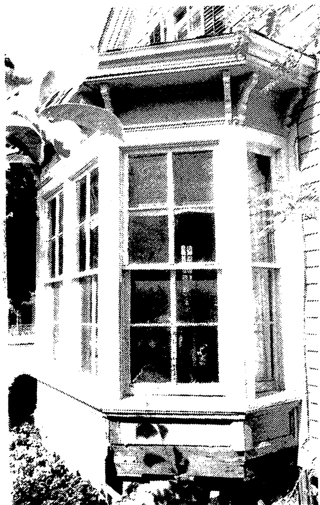
One side of the bay on a Washington Street home is under construction, needing major repairs; the other side remains undisturbed.
