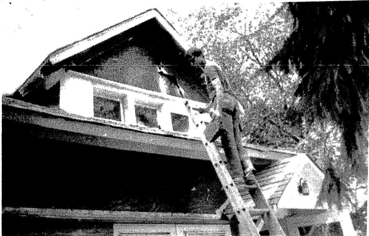
Restoration work on the Clarkston Conservatory of Music on Main Street proceeds with
