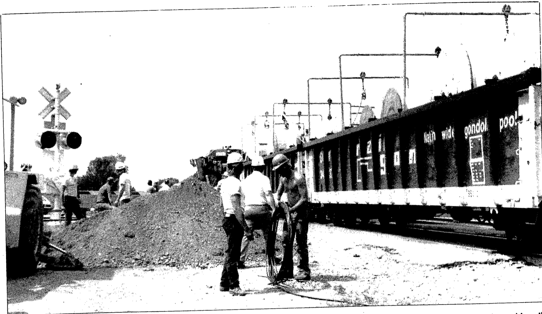
Traffic is stopped periodically so the five-car construction equipment can make its way
