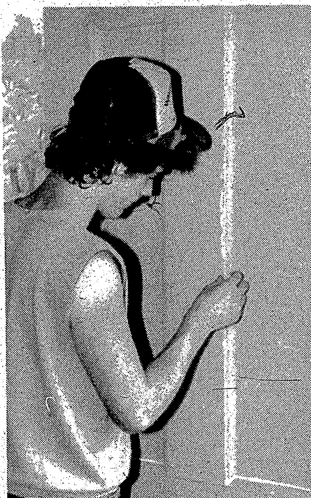
Time is taken to fill in the tiniest cracks.
