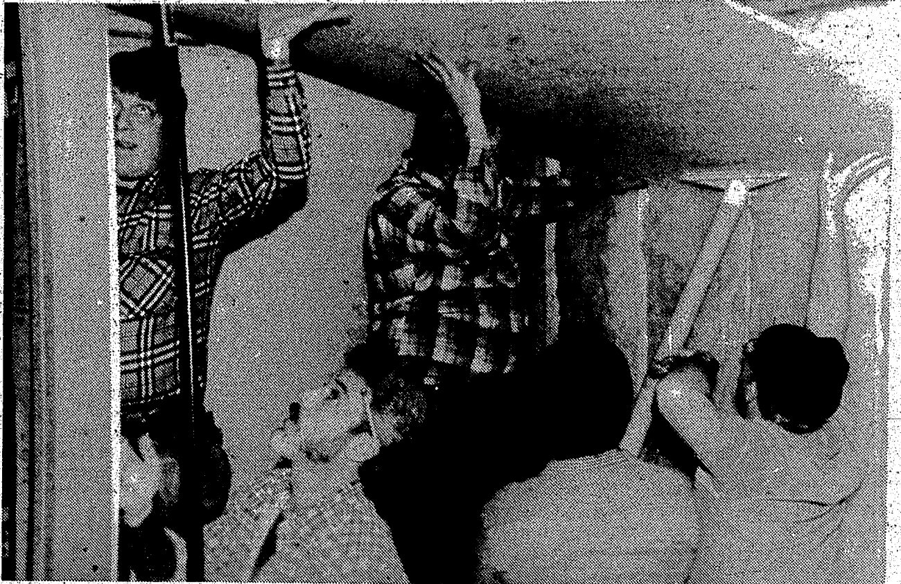
Tight quarters prevail as volunteer workers put up the ceiling above the women's room under construction at the Depot Theatre. From left
