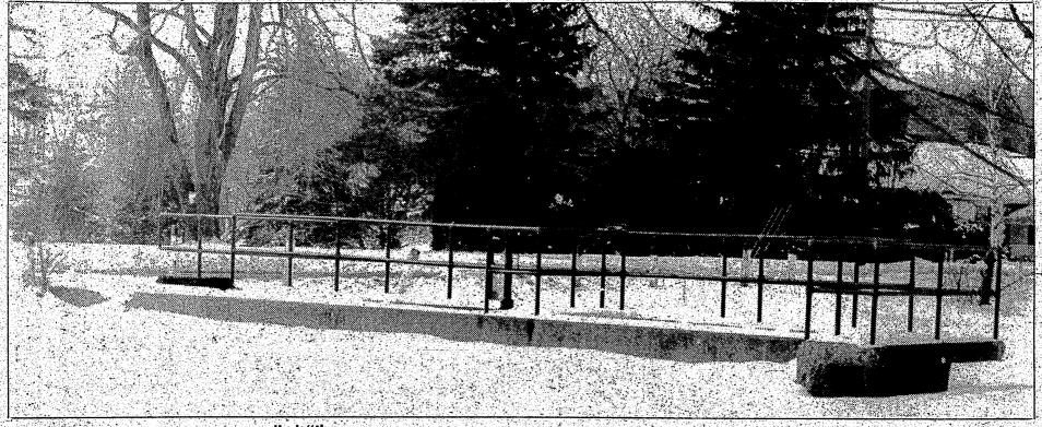
This cement and metal structure called "the hydro" was built off Washington Street into the Mill Pond by Henry Ford. It contains power works that serve to control the water flow under
