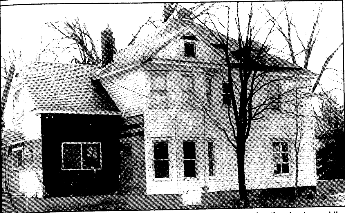
exterior of the house is the summer project the Hudsons. They started on the outside last summer by removing the aluminum siding and the rotted eaves.
