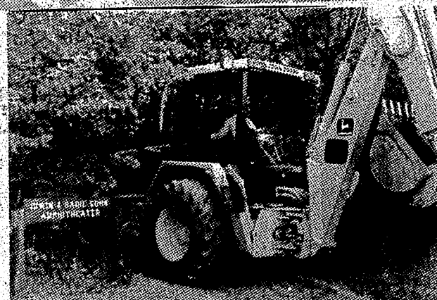
John Sowels drives a backhoe carrying topsoil down the path to the amphitheater. When work is completed, sod will cover the soil.
