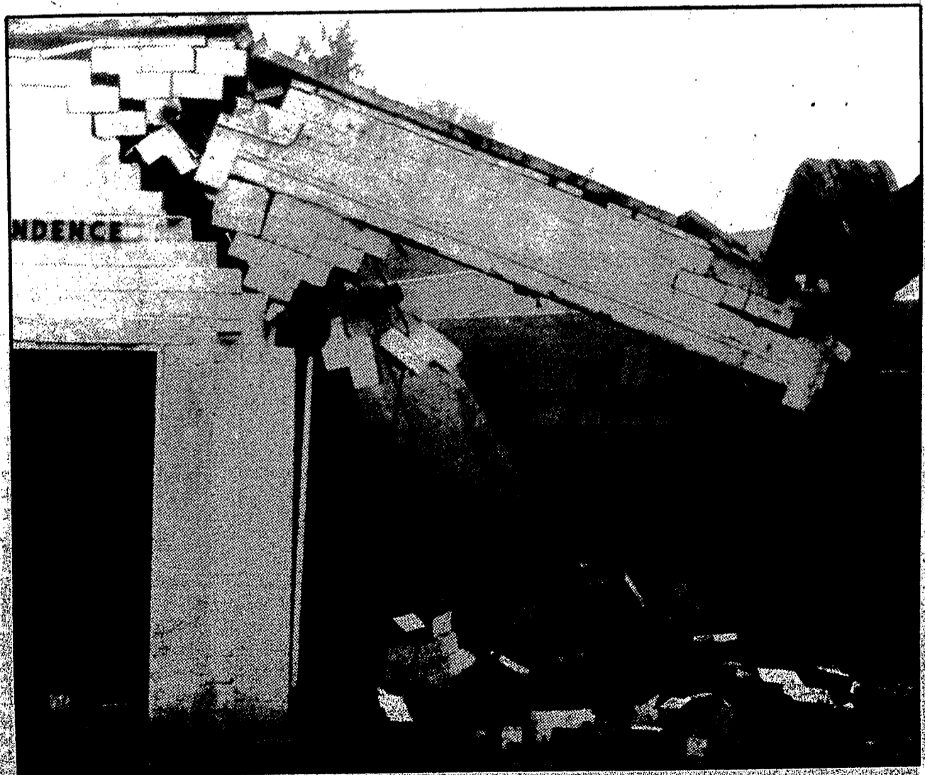
THE BUILDING that housed Independence Township Fire Station 2 for 33 years came down June 2 to make way for the new station at Sashabaw and Clarkston roads.
