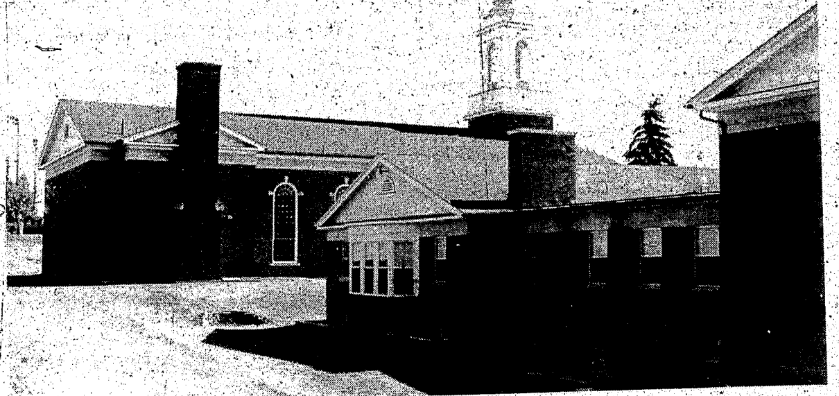
A NEW ADDITION to the Clarkston United Methodist Church at 6600 Waldon Rd. was completed recently, and consecration activities are set for Labor Day weekend, Sept. 4-5.
