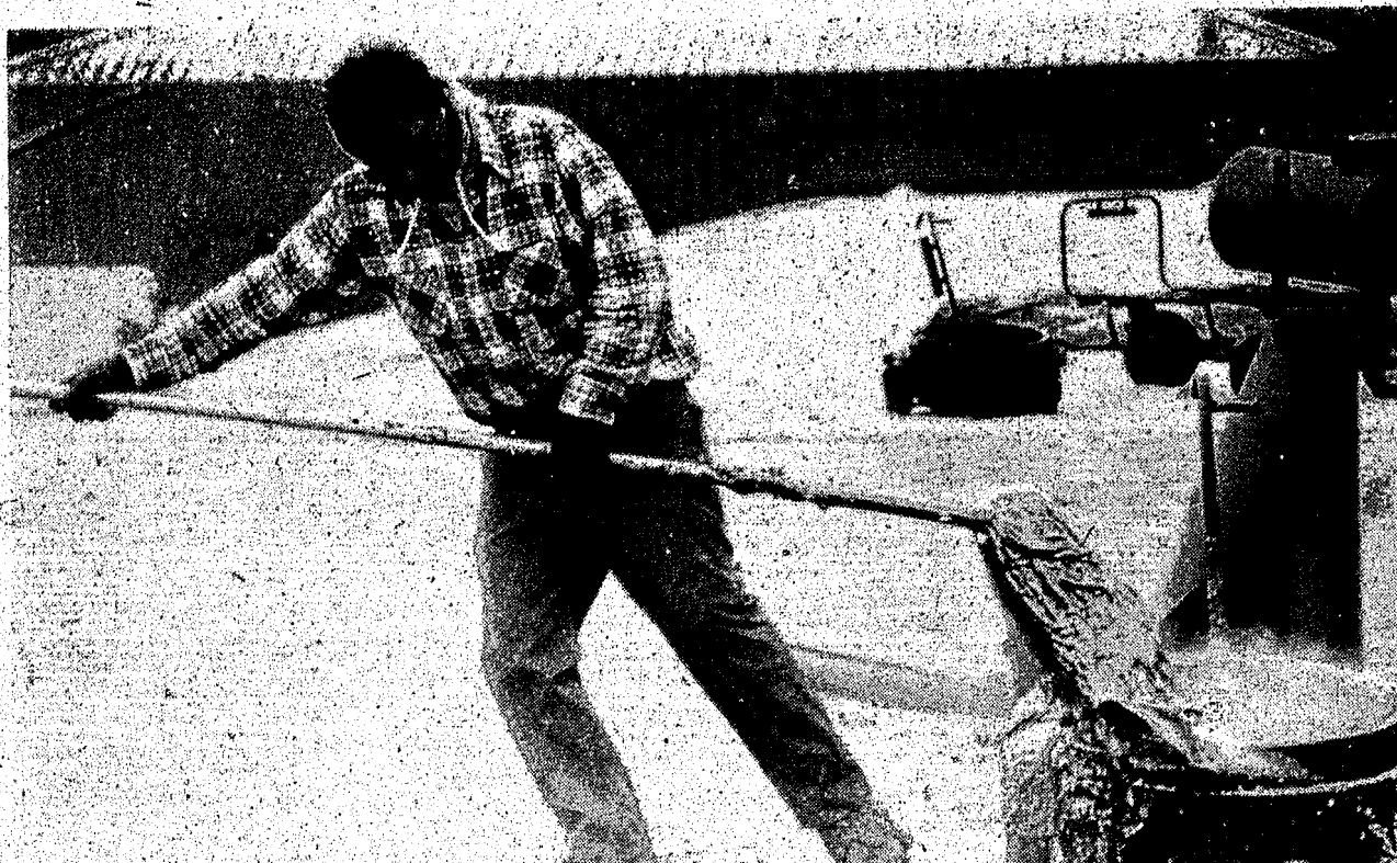
UP ON THE ROOF: As a dozen workers complete the variety of roof replacement tasks at Pine Knob Elementary, Jerry Hudak mans a 100-pound mop dipped in 400-degree tar.
