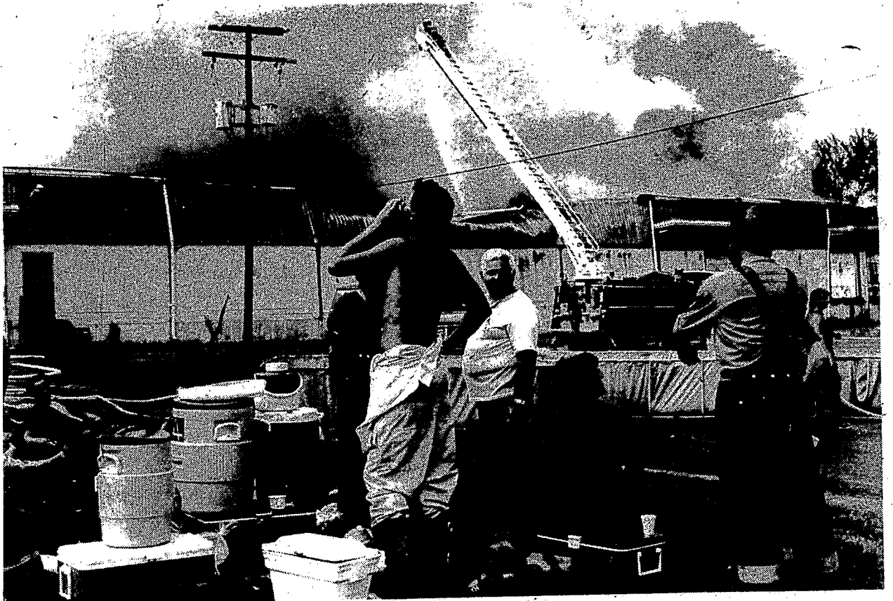
AFTER THE FIRE at Tra-Tech Midwest is under control, firefighters cool down. The fire completely destroyed the Dixie Highway building. (File photo by Kathy Greenfield)
