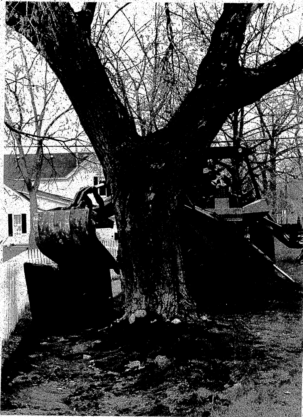
MANEUVERING A BACKHOE between fence and trees on Robertson Court, Clarkston, proves to be no problem for Javier Ozuna. No damage was done to tree or fence.
