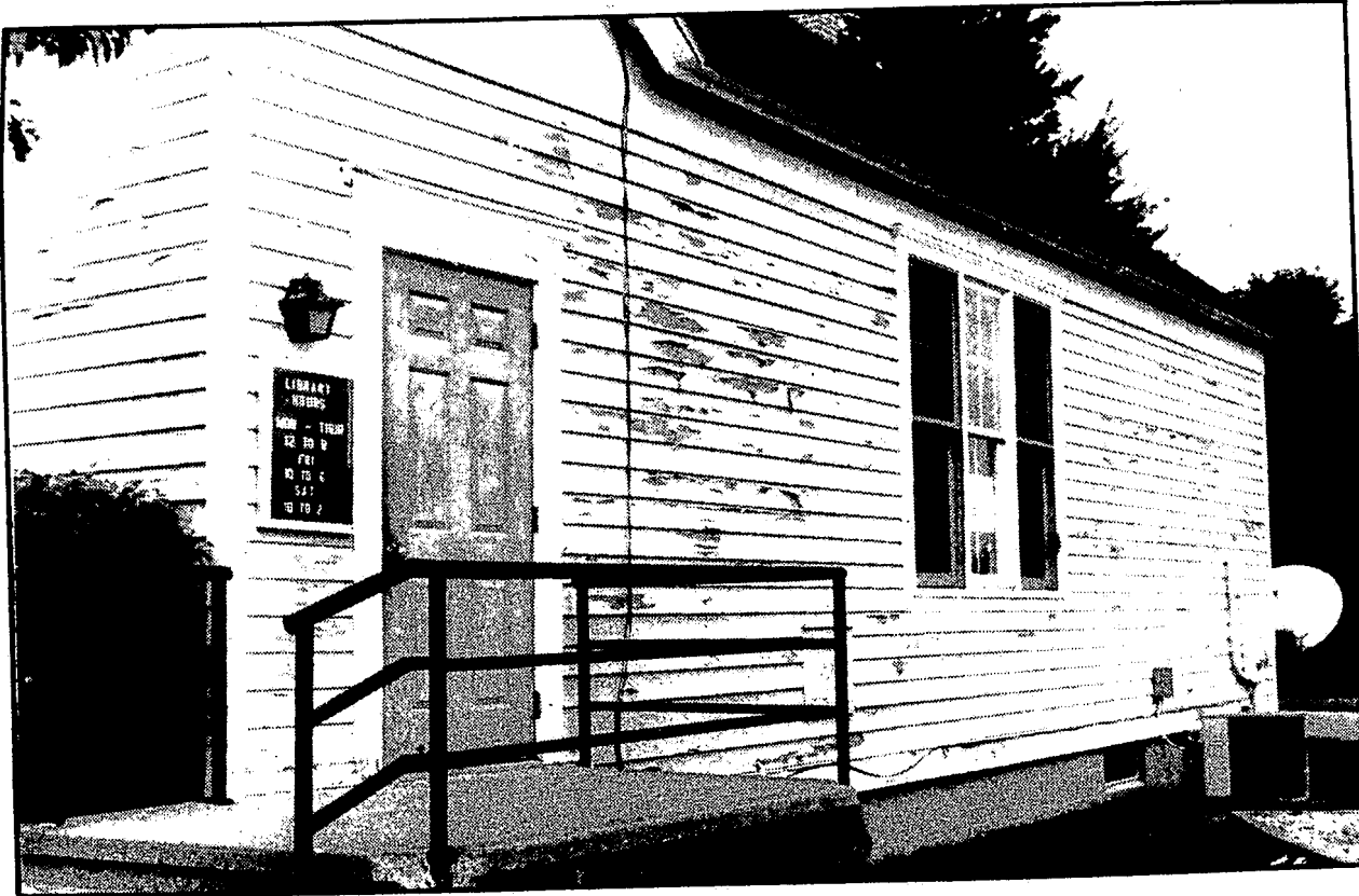
EVEN AFTER a recent painting, the Springfield Township Library paint is peeling on all
