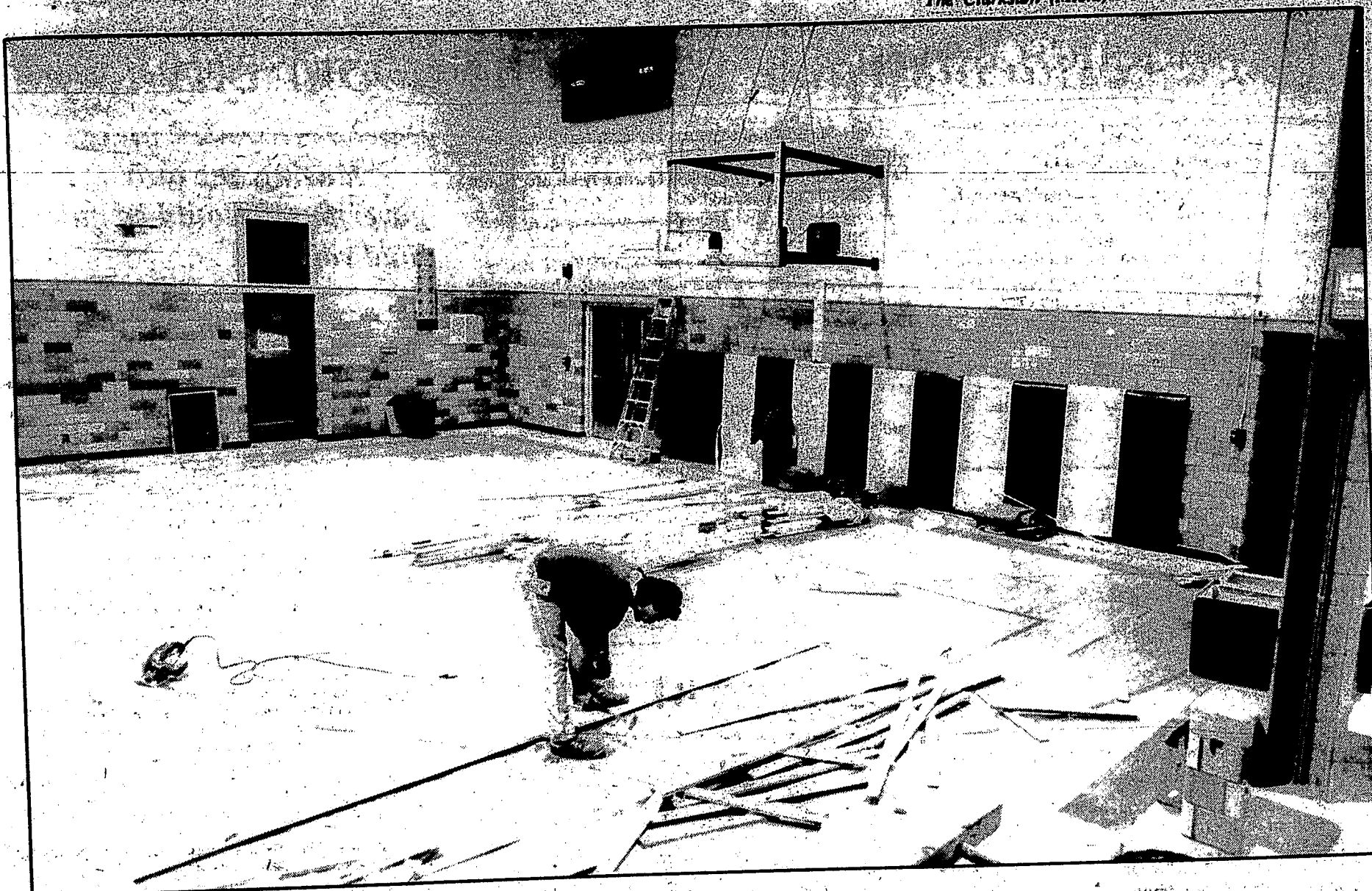
DEAN Ruffolo of the Remington Floor Co., Melvindale, works on the Clarkston Junior High School gymnasium floor Feb. 19. Repairs include sanding and sealing plus
