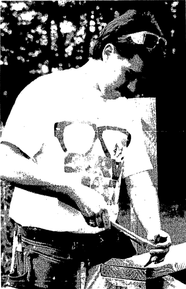
CHRIS MERZ, 17, prepares one board for its spot in the new wheelchair ramp.
