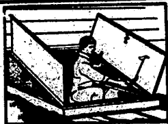
Secure to concrete and caulk.
