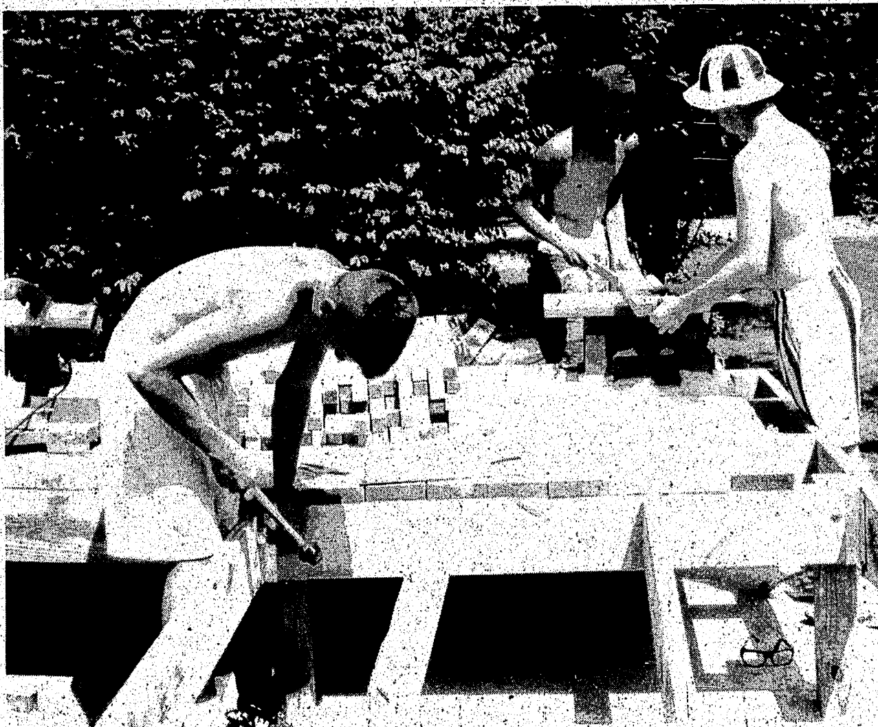
WORKING on the Woodys' wheelchair ramp are (from left) Guy Myers, Paul Zink and Matt Marcell. The volunteer teens worked for a
