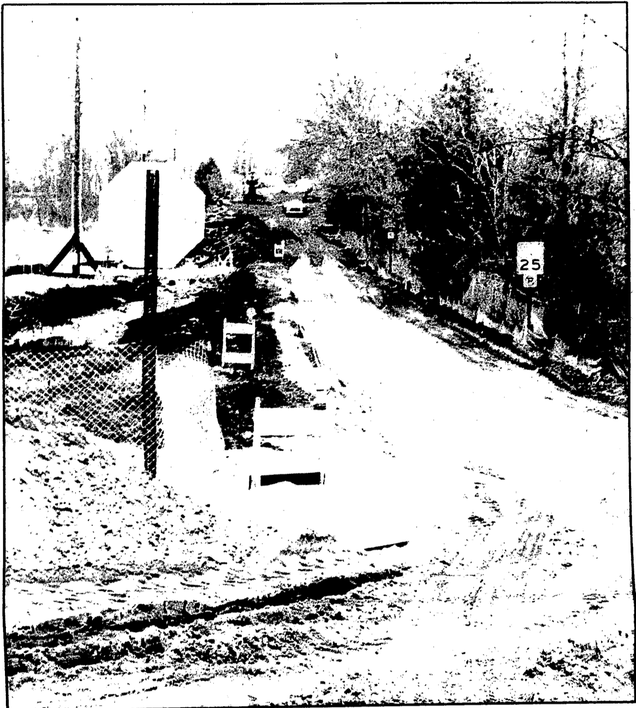
DEER LAKE Road is closed at least through March 6 to allow for sewer construction, according to Mel Vaara. Clarkston school
