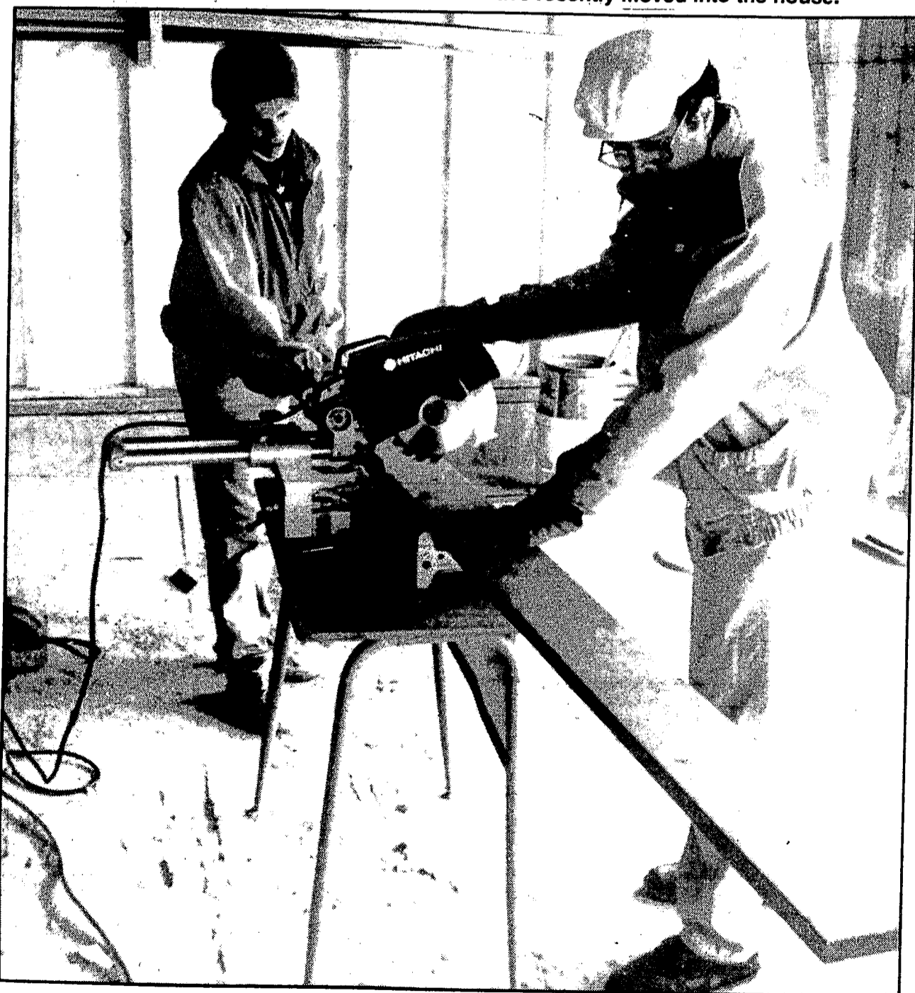
WATERFORD Kettering High School Junior Matt Gilboe, left, and George Howard Jr. with the Phase II program from General Motors make sure they make the correct cut.
