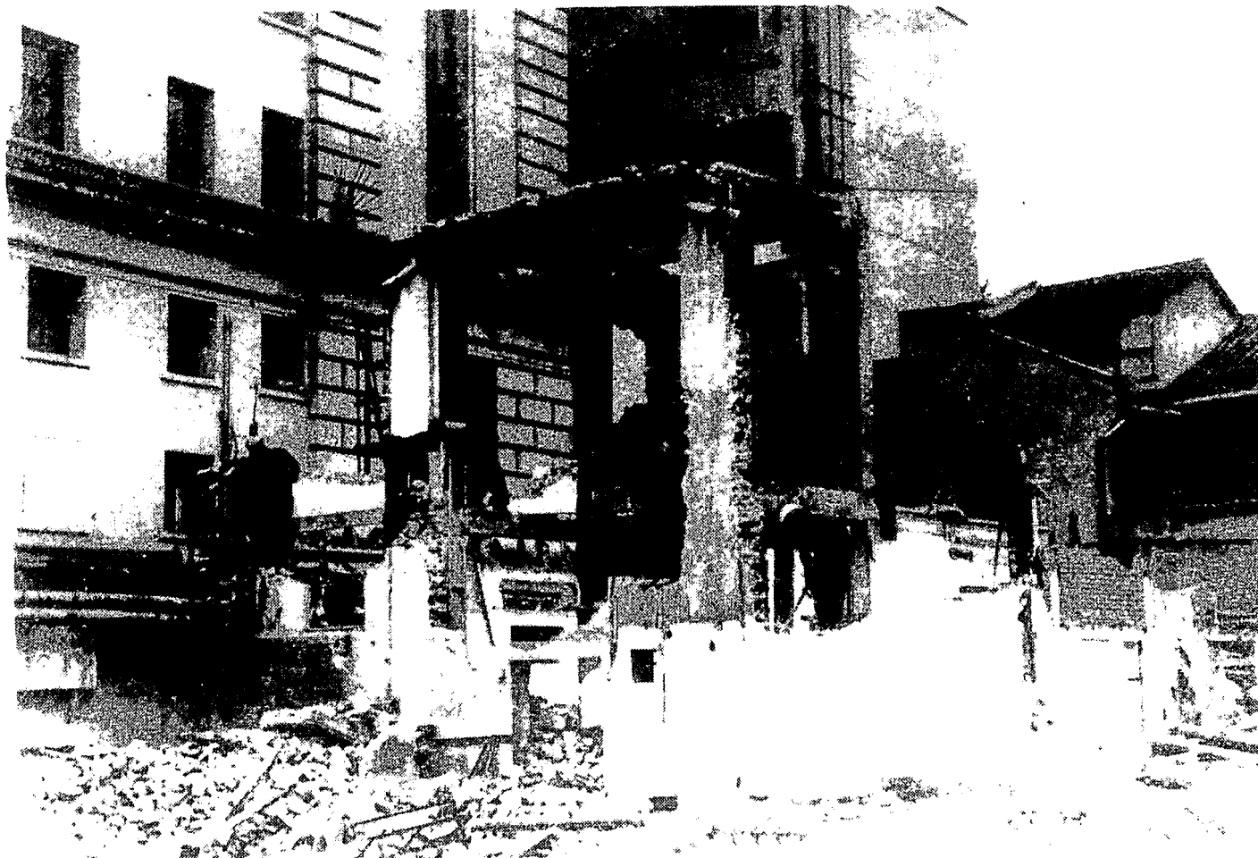
All the buildings we saw being demolished were done with sledge hammers and crowbars. Old streets were being torn up the same way.
