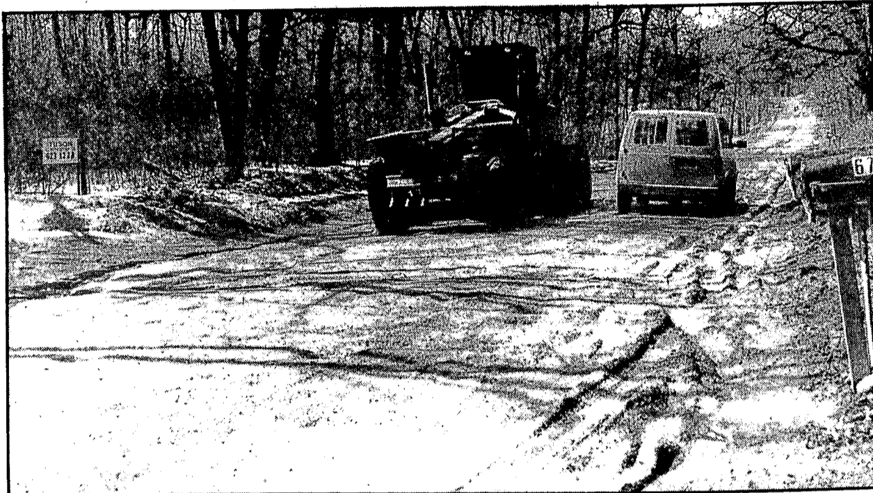
WHEN WARM weather hits, the Road Commission for Oakland County bumpy grades gravel roads in the area. Here, Rod Pierson
