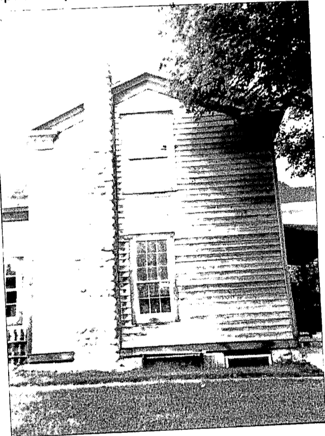
THE new stone chimney, made from foundation stones, gives the parsonage a more rustic look.
