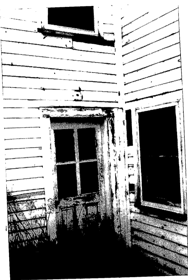
THIS PHOTO shows the private entrance to the apartment before construction and renovations began.
