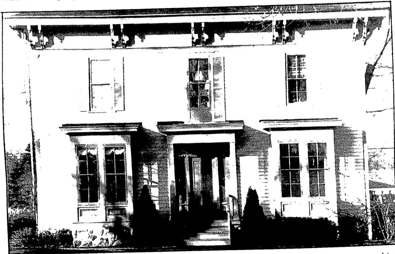
THE BOX-LIKE or cube with wide roof eaves supported by the large curving brackets characterize this Italian Revival home on
