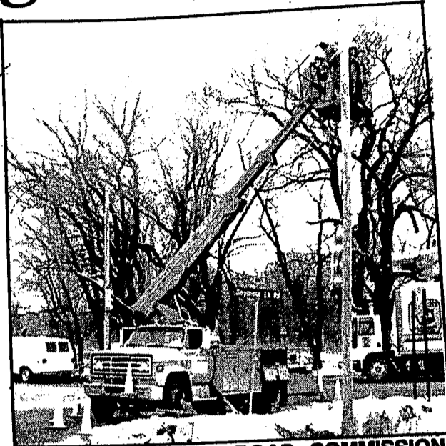
OAKLAND COUNTY ROAD COMMISSION WORKERS began the full-day process of installing a new signal at M-15 and Seymour Lake roads last Friday.
