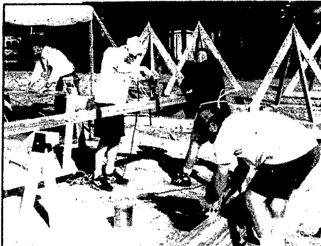
Workers sweated through record heat to get the playscape completed.
