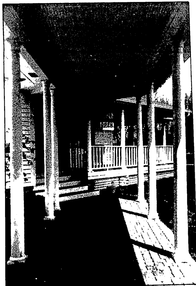
This side view of the outside features a covered walkway leading to a side door. The sign gives a hint to what's inside the door—the kitchen.
