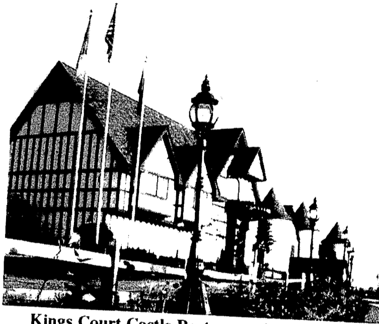
Kings Court Castle Restaurant is located in Olde World Canterbury Village (810)391-5780
