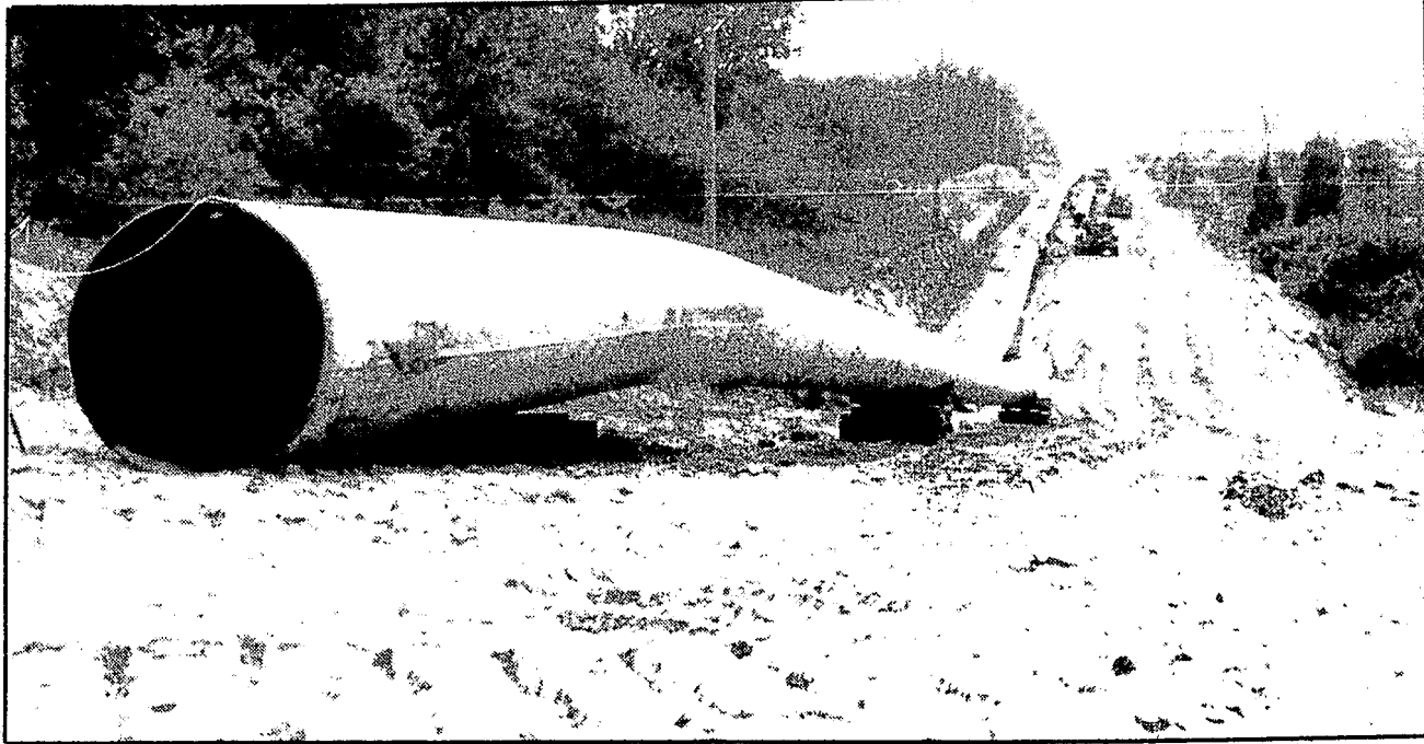
Workers begin the process of welding the pipes together at a section of the pipeline on Teggerdine
