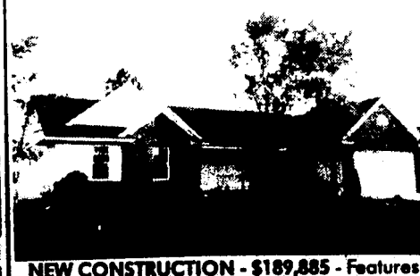
NEW CONSTRUCTION - $189,885 - Features paved streets, natural gas, sewer & water. Full basement, 1600 sq. ft., 2-1/2 baths, hardwood floors, white cabinets, great room with fireplace. Also includes sprinkler system & landscape yard. Lapeer West schools. L3791WE
