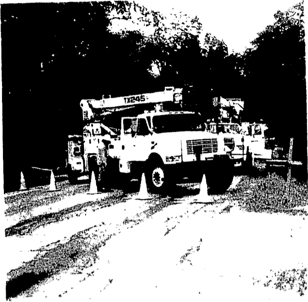
Detroit Edison workers closed Clarkston Road west of Sashabaw for several hours Sunday after high winds knocked a willow tree down on top of power lines.
