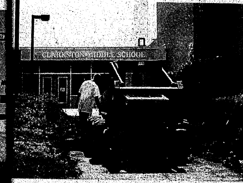
The main entrance to the new Clarkston Middle School (old CHS). Interior finishing and cooling nears
