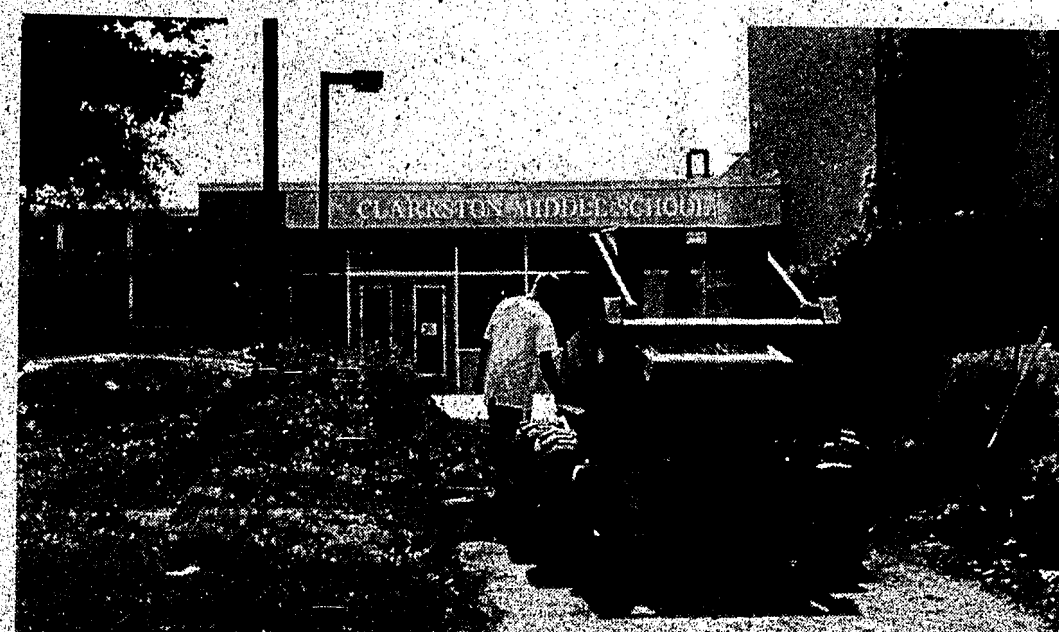
Workers prepare the main entrance to the new Clarkston Middle School (old CHS). Interior finishes continue, heating and cooling nears
