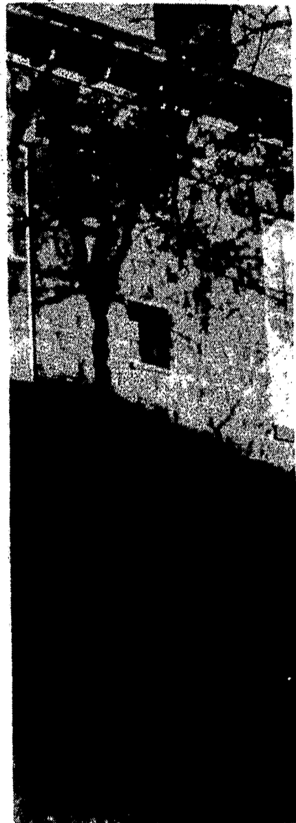
Vandals gained entrance to the Clarkston Branch of the U. S. Post Office by forcing the small window in the center of the picture. Marks indicated that a ladder was probably used to reach the window.
