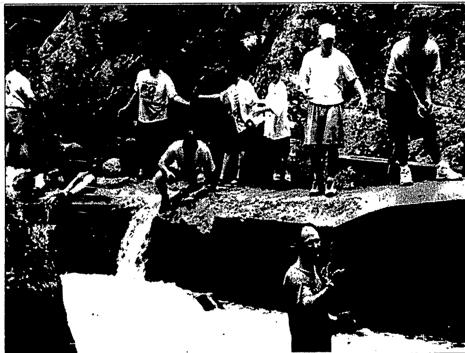
Members of Clarkston Community Church work to reroute a river so a dam can be built in Canchias. This was the church's first visit to Honduras.
